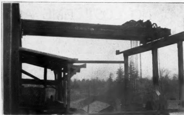
Traveling Crane Installed Over the Crushers
